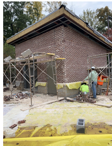
CSK- Storage Building Brick Install
