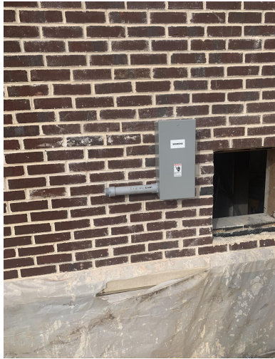
CSK- Electrical Disconnect Install
