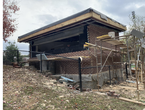
CSK- Storage Building Brick Install
